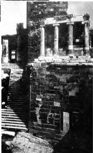
Fig. 7.40. A close-in of a fragment of an old photograph dating from the 1860's. It is clearly visible that the mediaeval Ottoman tower and the "ancient" foundation of the Athena Nike temple have identical masonry and are built of the same kind of stone. These constructions obviously belong to the same epoch. Taken from [198], page 39.
